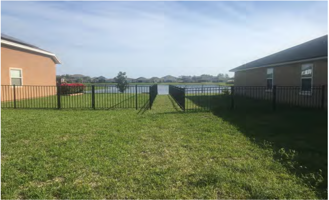
Downing Creek Drive (fencing encroaching on a 15' unobstructed drainage easement)(4-5-2018)
