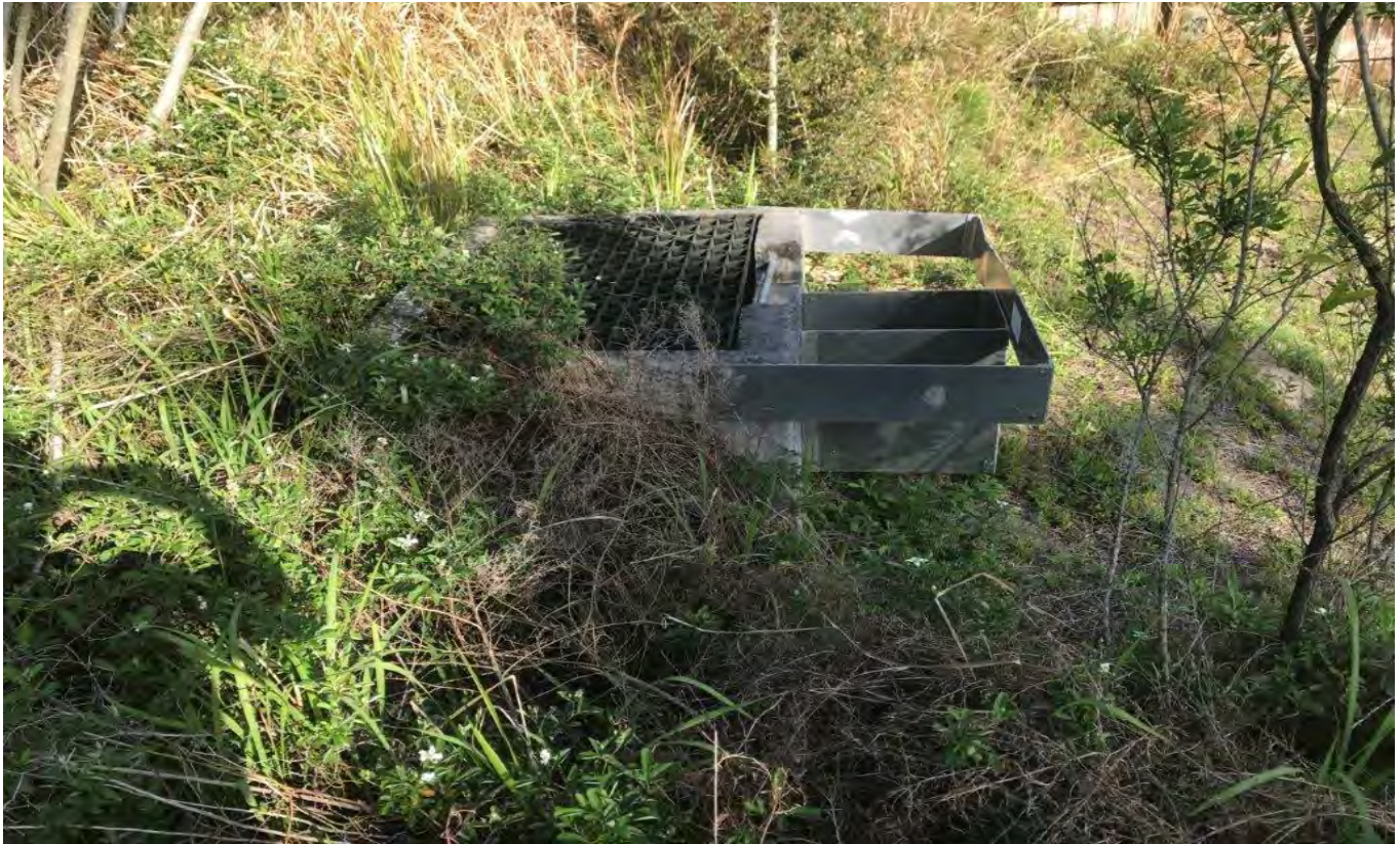
Smf 8 – Control Structure – Overgrown with weeds etc. (facing Westerly) (4-5-2018)
