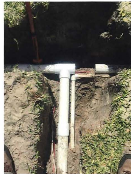
Irrigation line break at sports field
