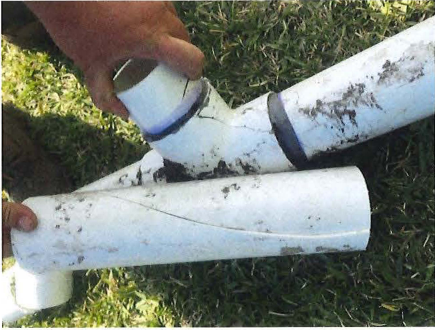
Cracked irrigation line – from vehicle traffic
