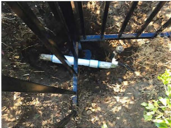
Irrigation line break during installation of new pool fence
