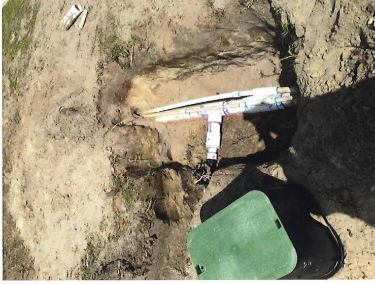
Adding irrigation valve to field
