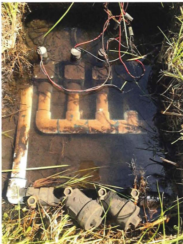
Broken irrigation manifold in old pocket park
