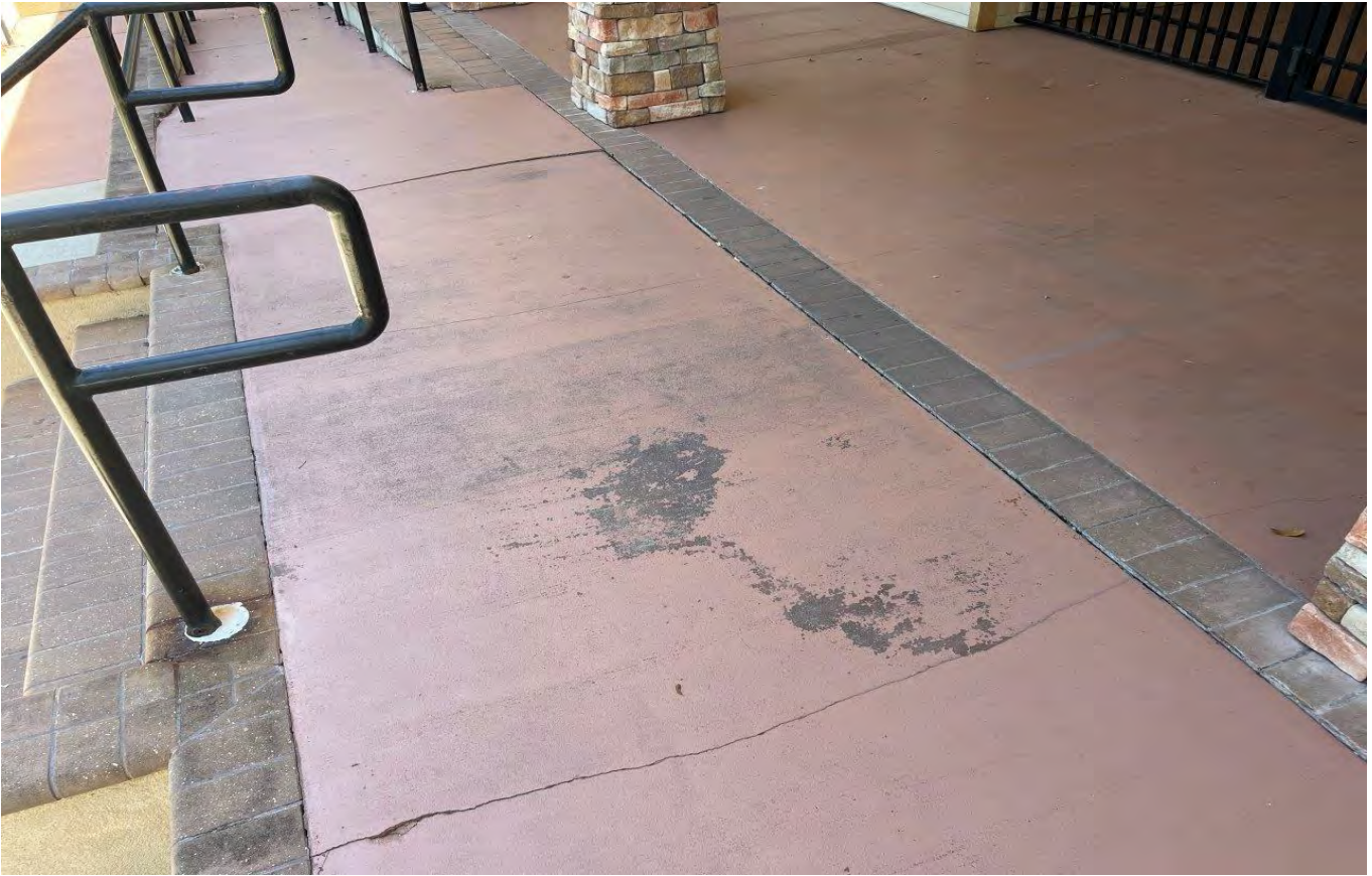
Amenity Center – concrete cracking (near front gate) (7-13-21)
