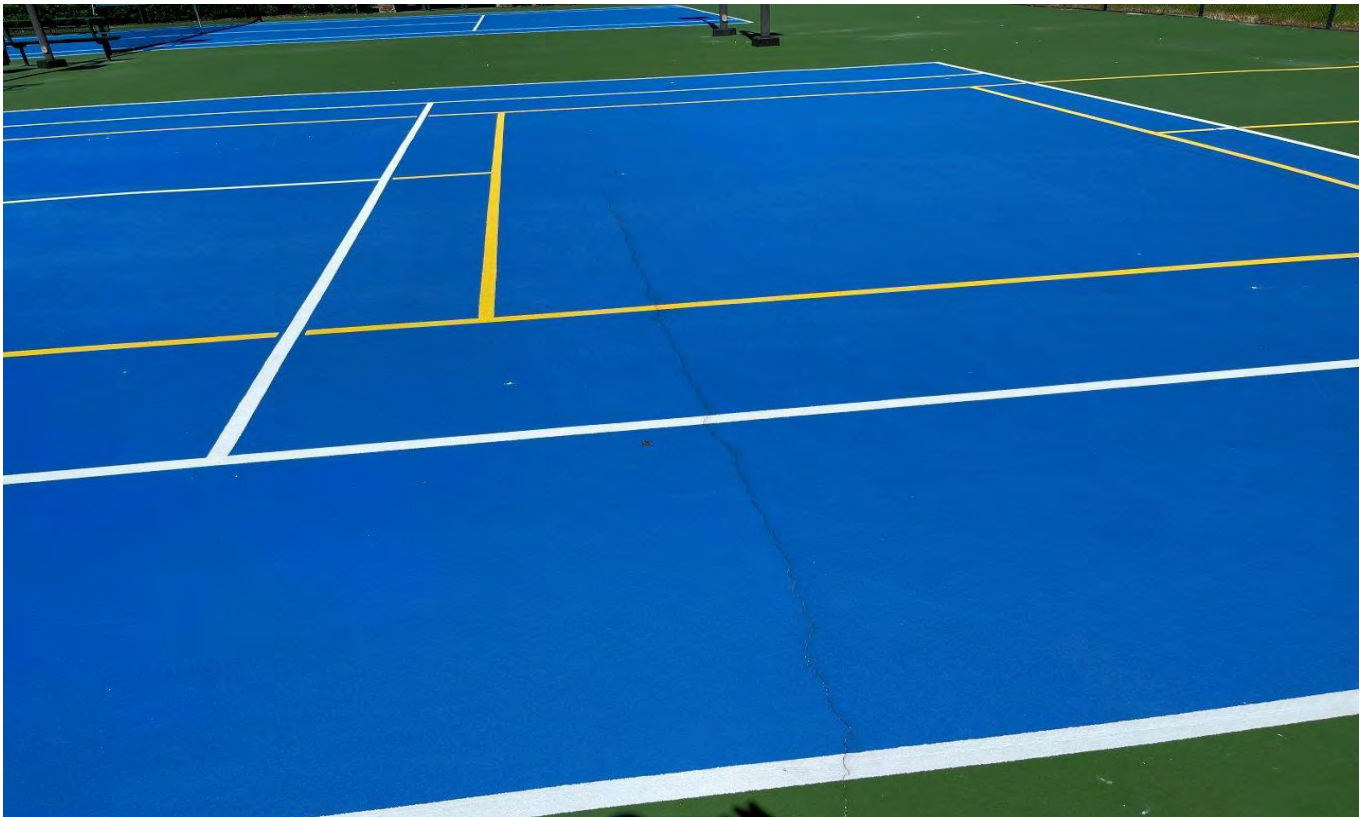
Amenity Center – Tennis Court (Minor Cracking) (7-13-21)
