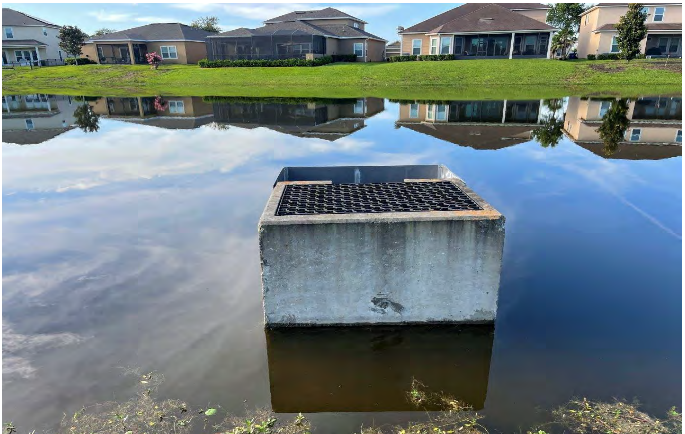
Storm Water Management Facility 7 - Control Structure (7-13-21)
