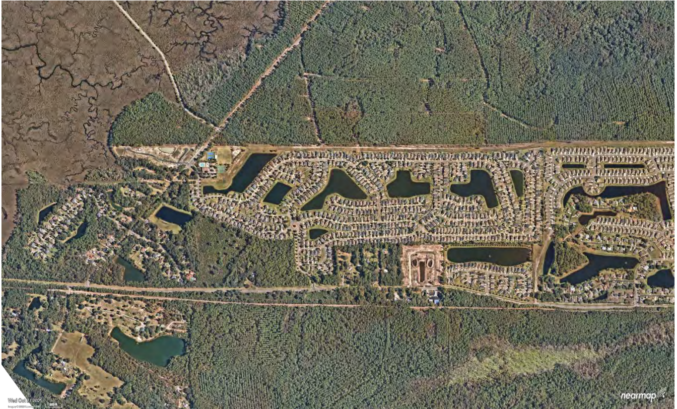
Aerial of Project (By NearMap) (Taken on 10-27-2021)
