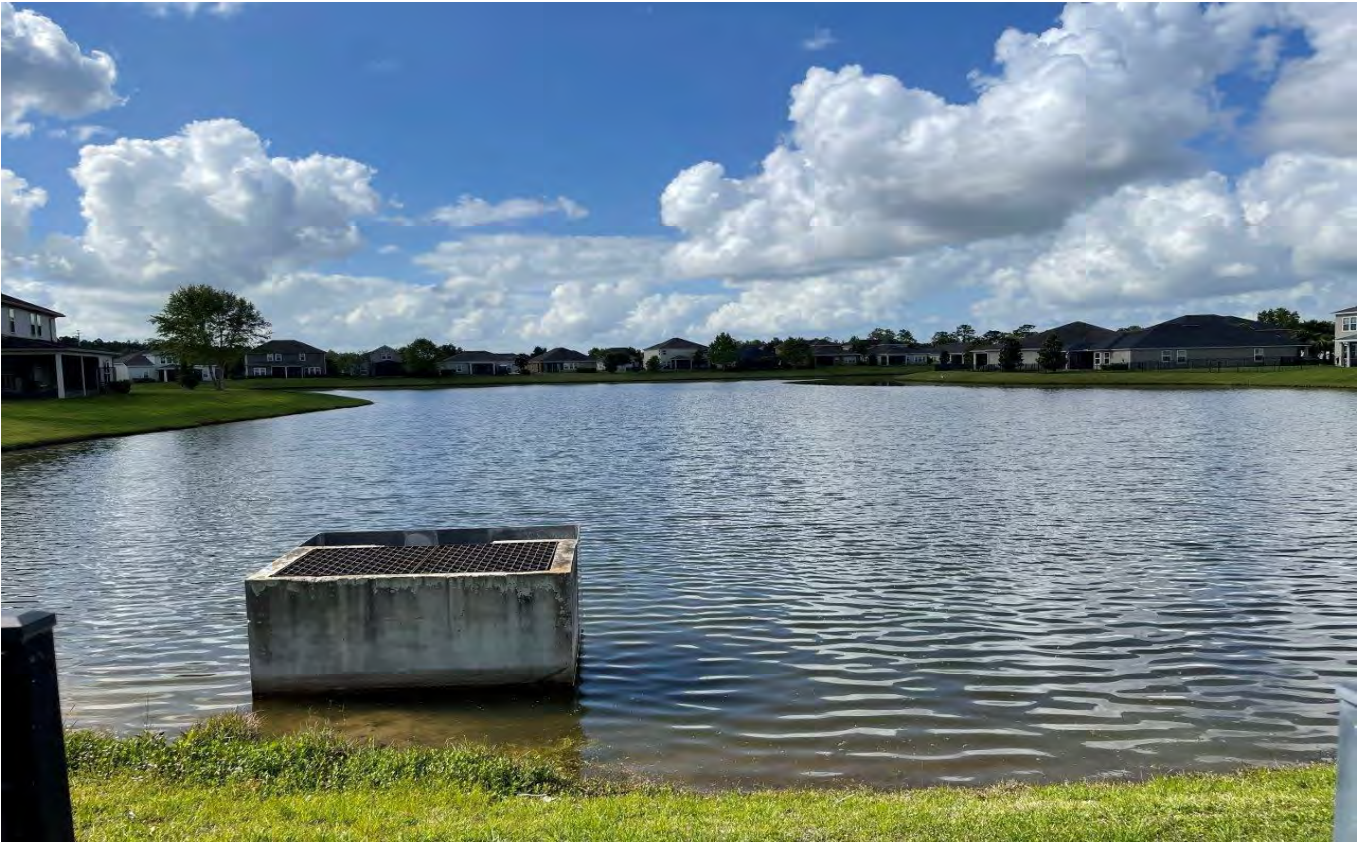
Storm Water Management Facility 6 (4-25-22)
