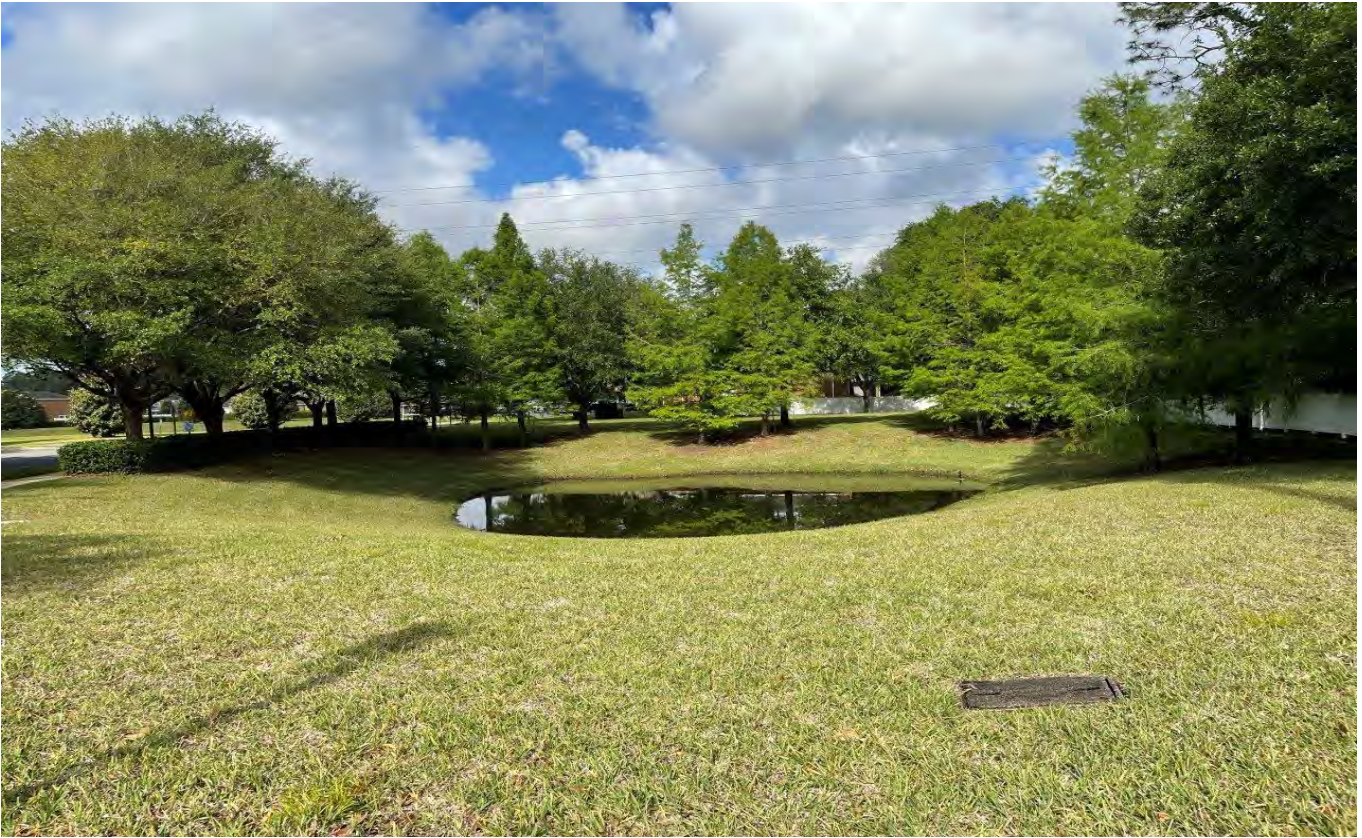
Storm Water Management Facility 9 (4-25-22)
