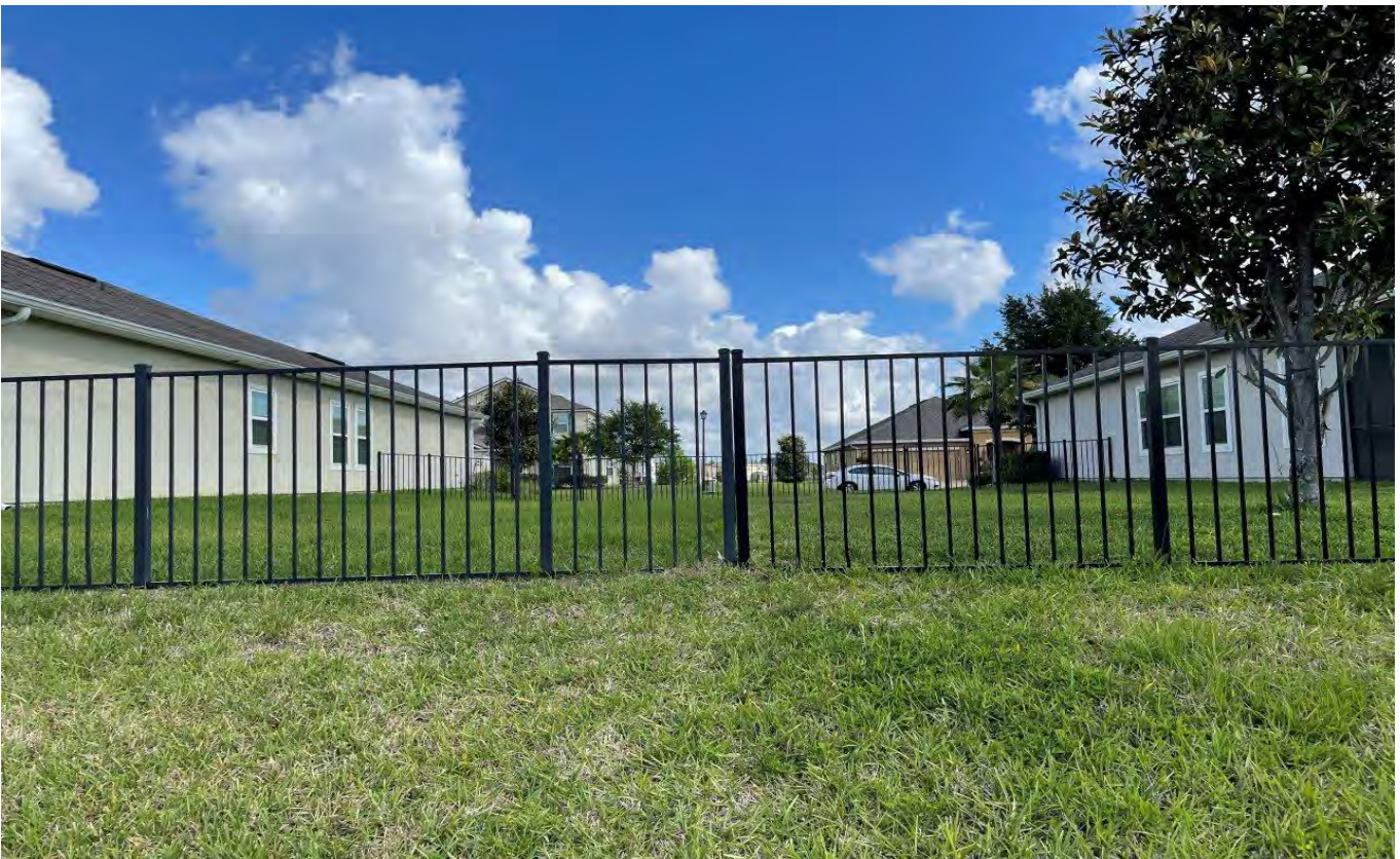
Storm Water Management Facility 7 Easement Access (Restricted) (4-25-22)
