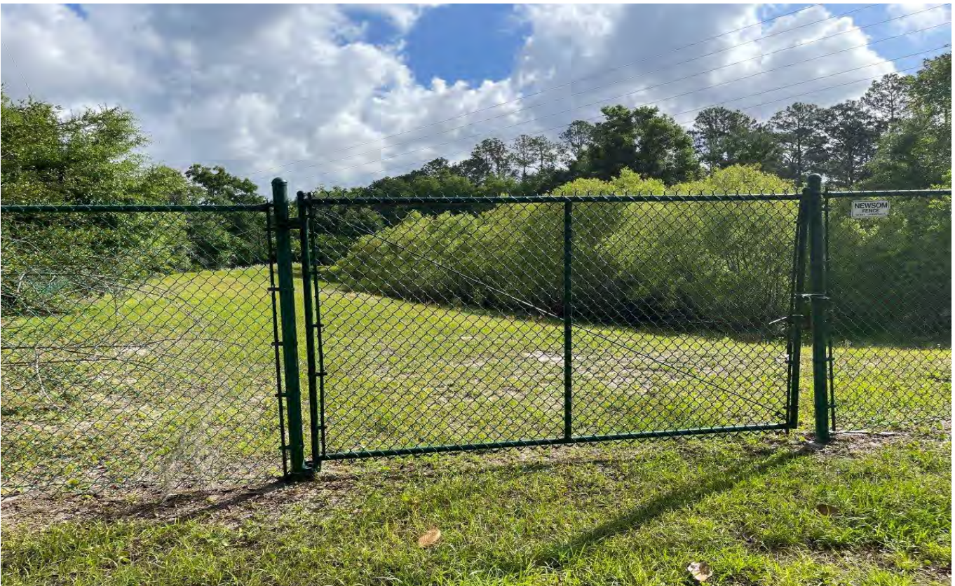
Storm Water Management Facility 8 – Gate Entrance (Owned by City of Jacksonville) (4-25-22)
