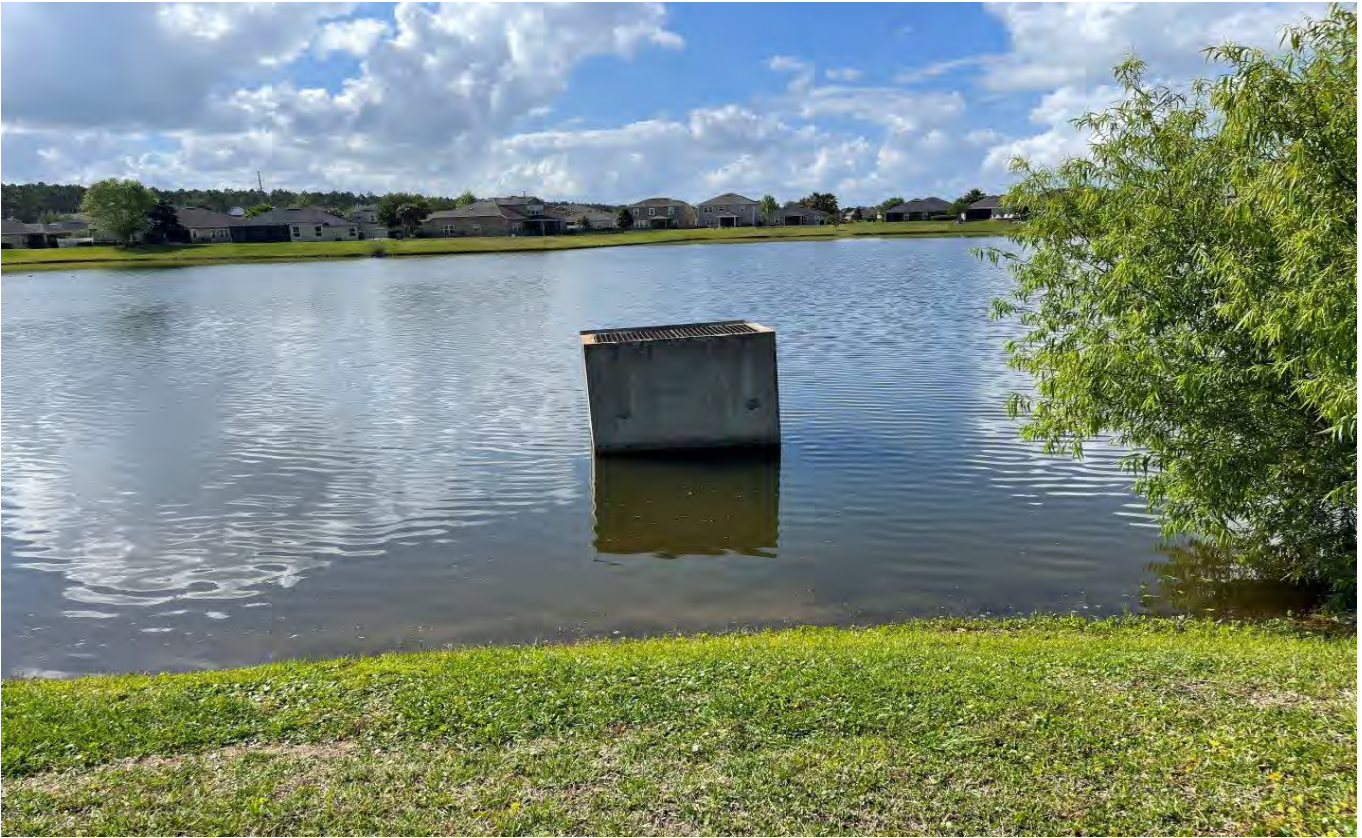
Storm Water Management Facility 5 Control Structure (4-25-22)
