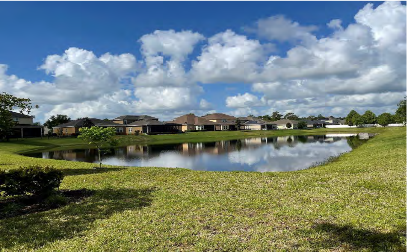
Storm Water Management Facility 7 (4-25-22)
