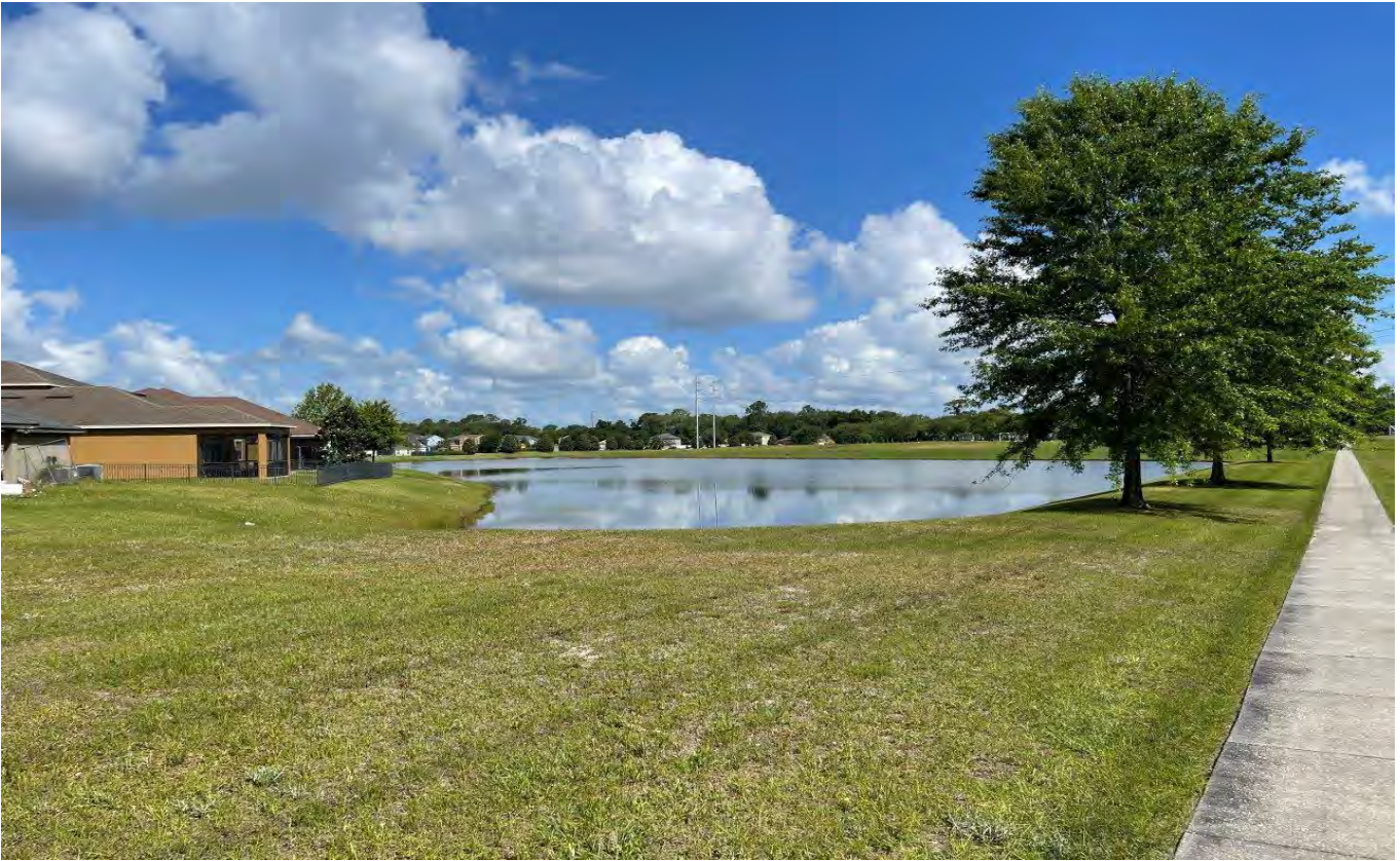
Storm Water Management Facility 1 (4-25-22)
