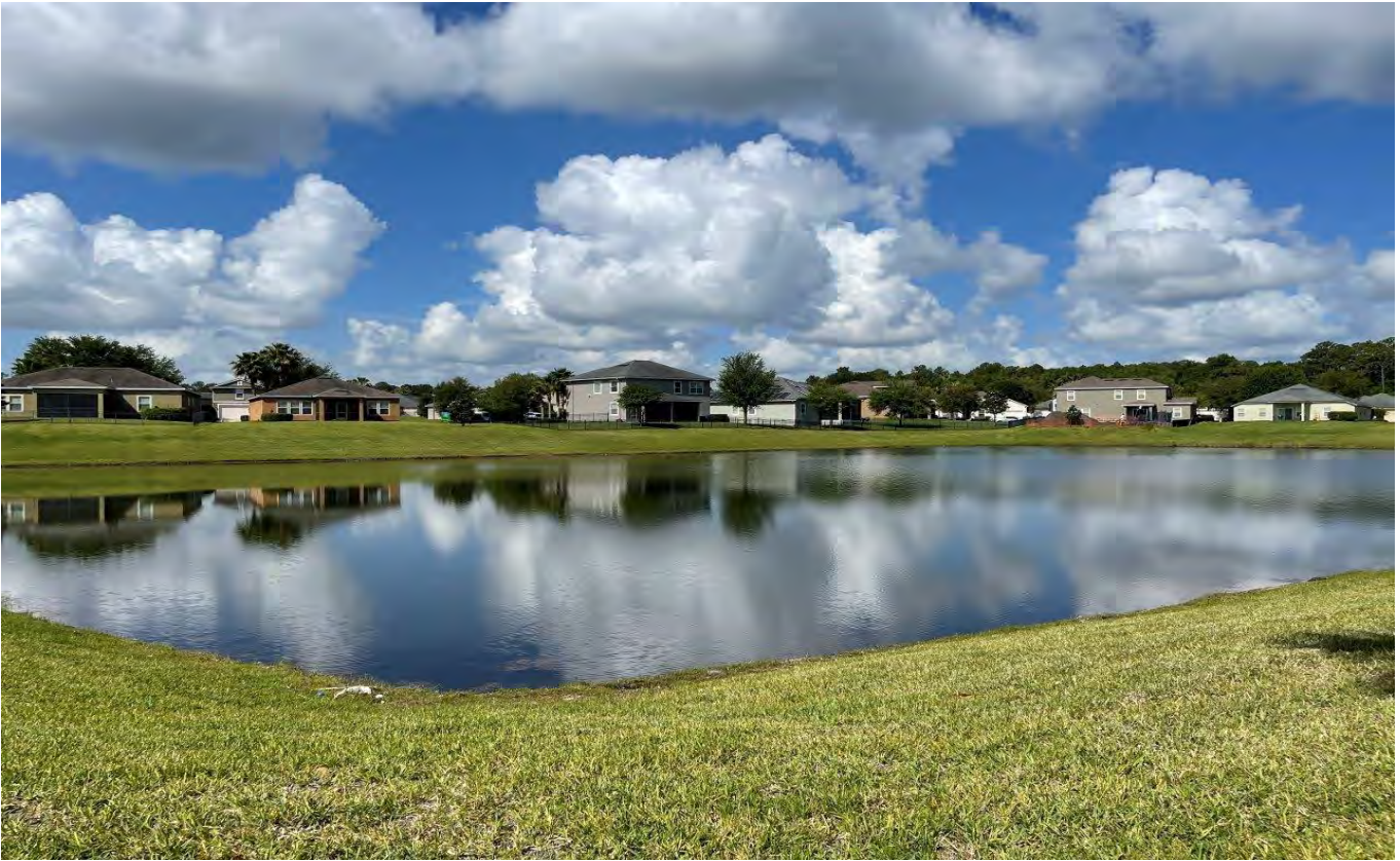
Storm Water Management Facility 2 (4-25-22)
