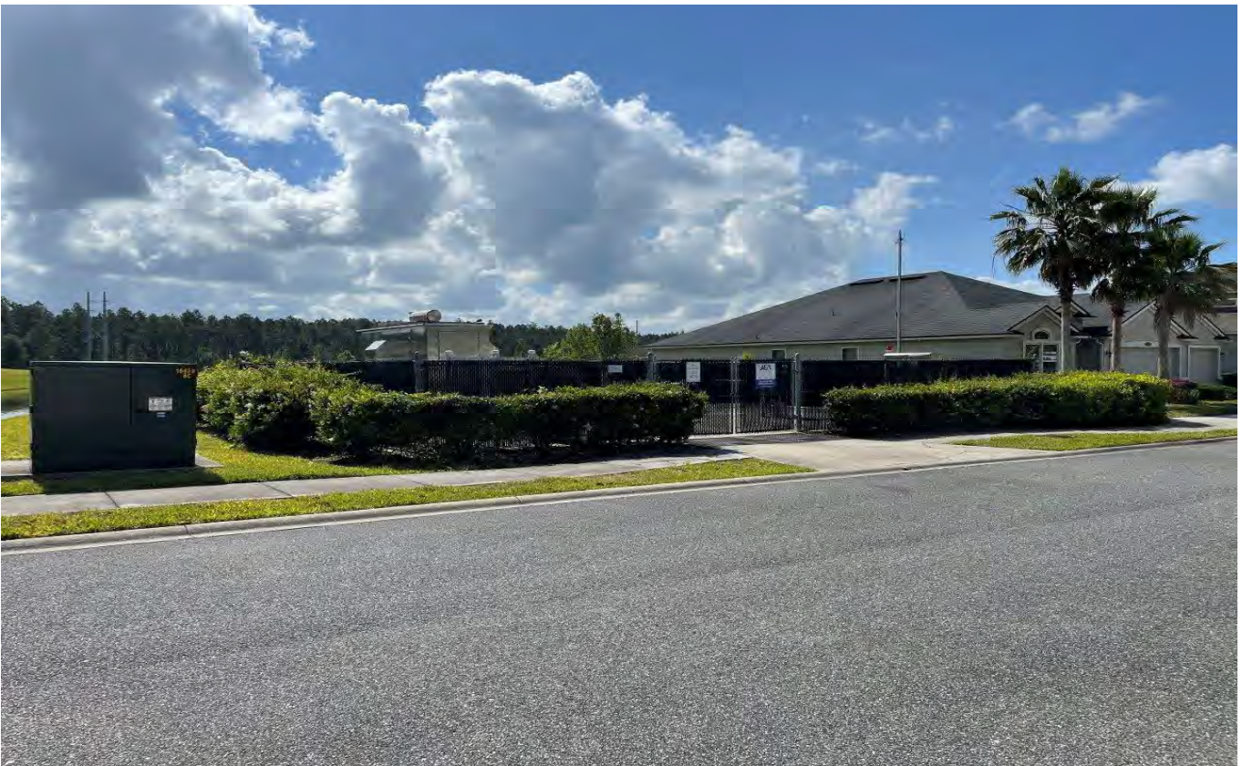
Lift Station – Landscaping (Maintained by the CDD) (4-25-22)
