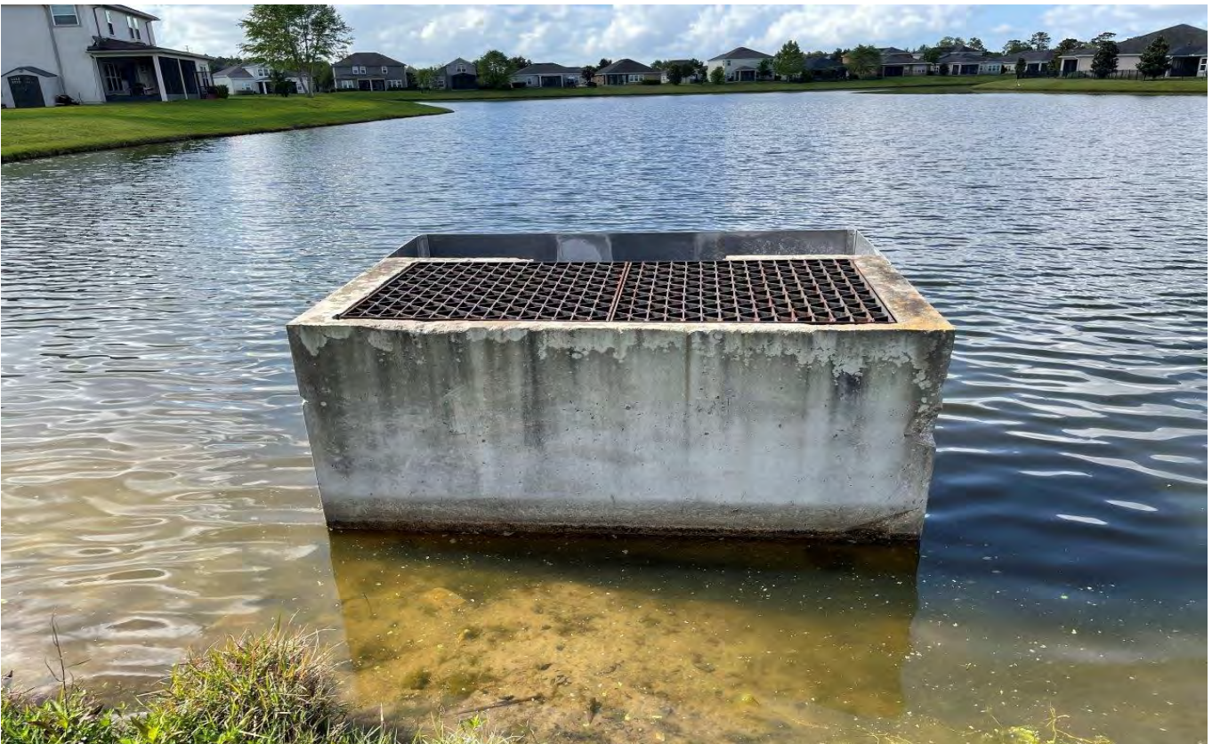
Storm Water Management Facility 6 - Control Structure (4-25-22)
