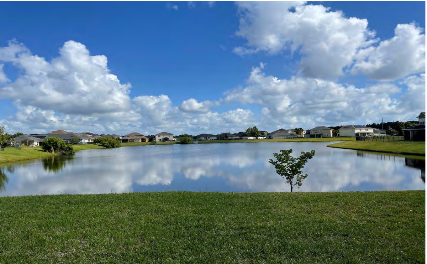
Storm Water Management Facility 5 (4-25-22)
