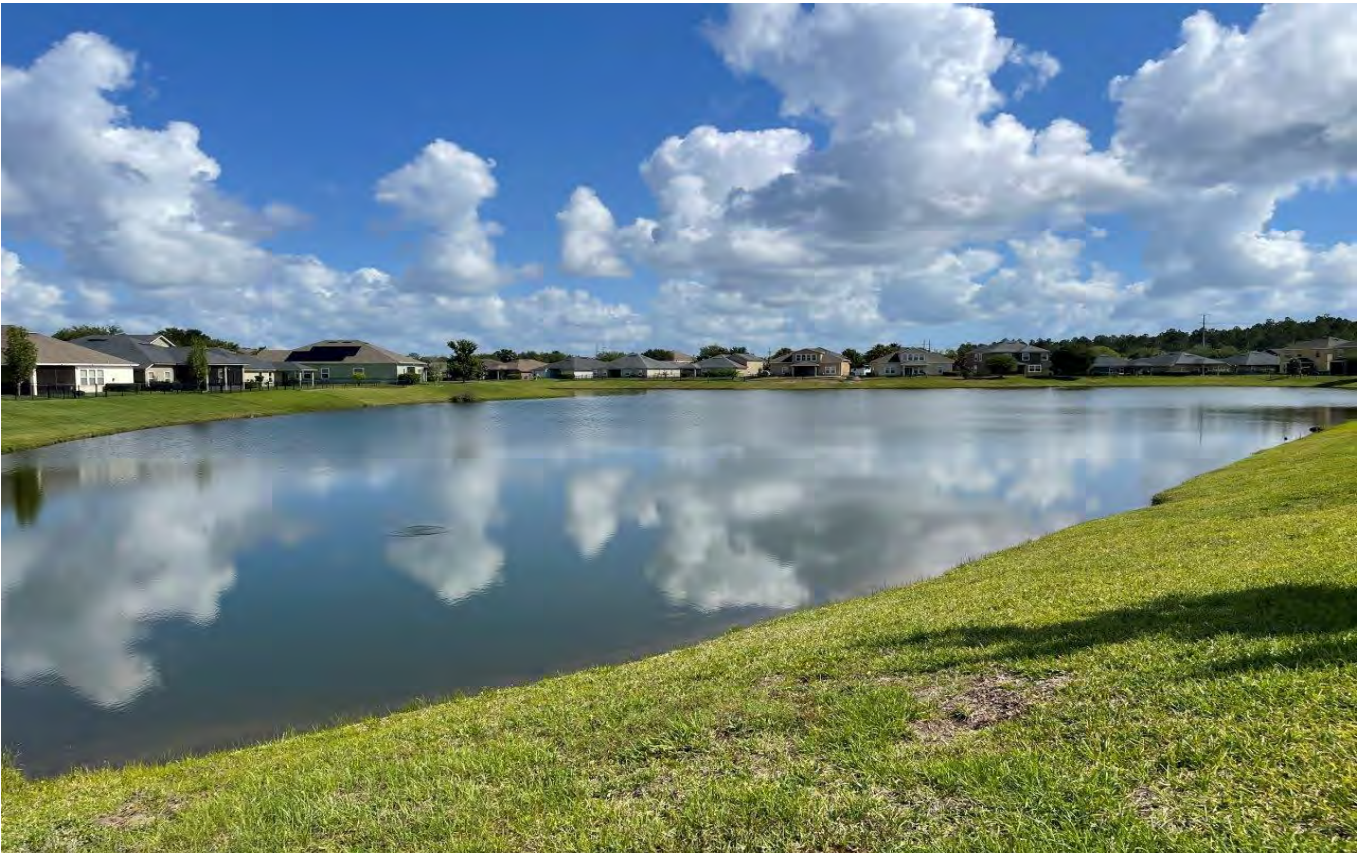
Storm Water Management Facility 3 (4-25-22)
