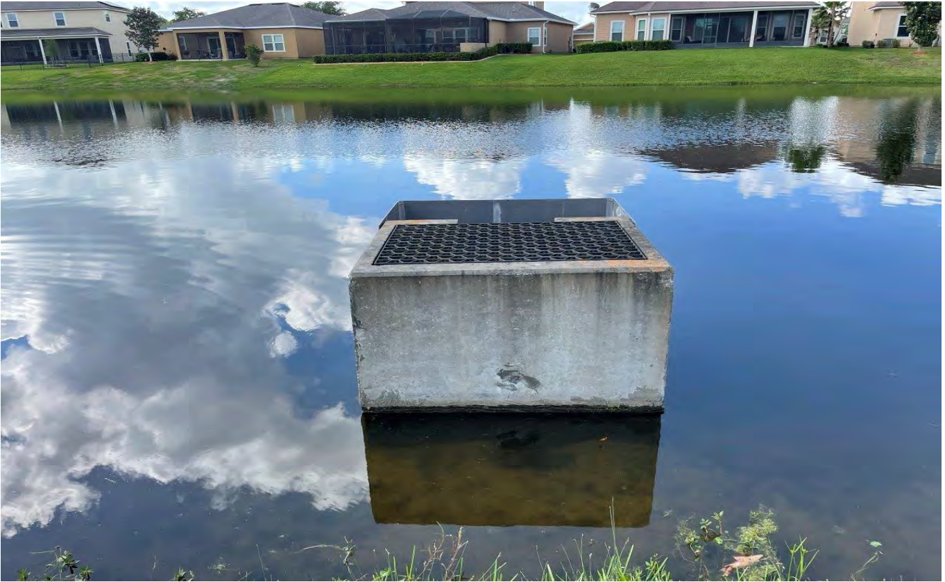
Storm Water Management Facility 7 - Control Structure (4-25-22)
