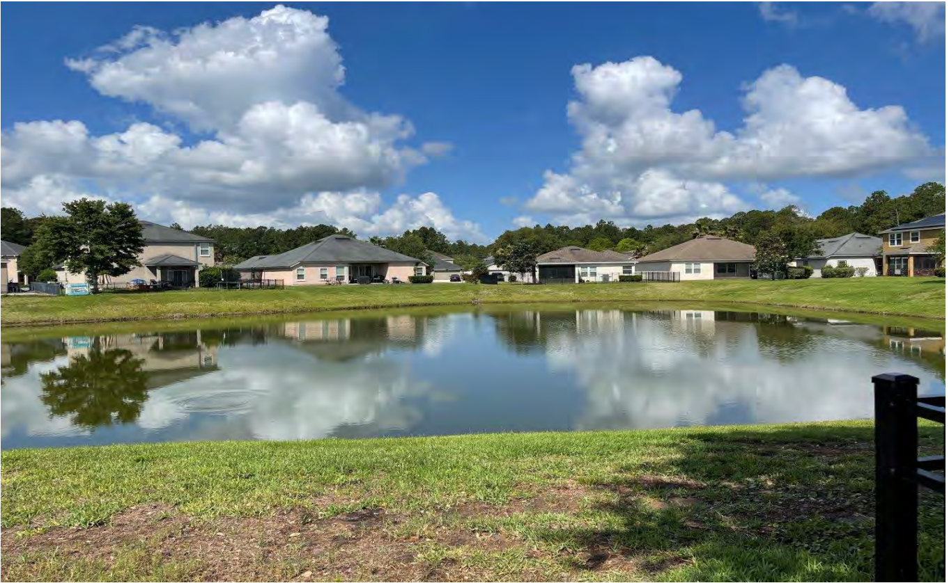
Storm Water Management Facility 4 (4-25-22)
