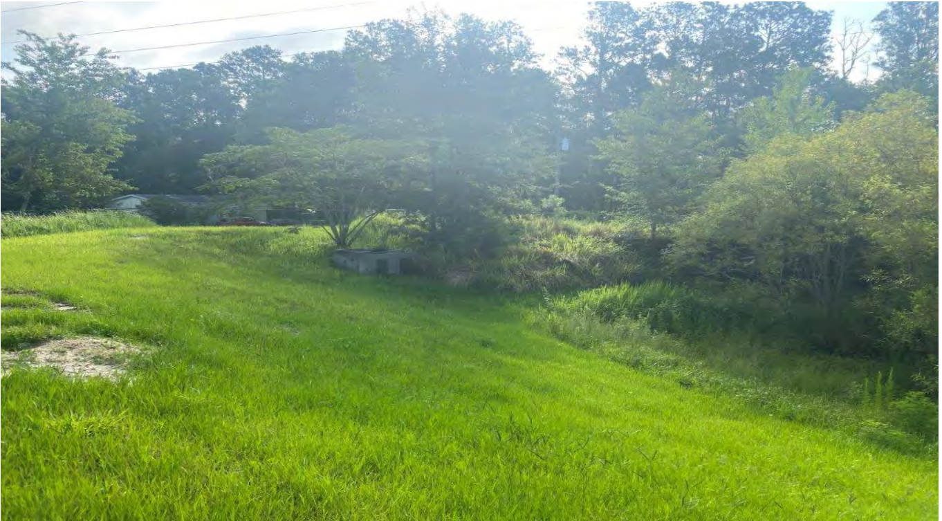
Storm Water Management Facility 8 – Gated Entrance (Owned by City of Jacksonville) (6-27-23)
