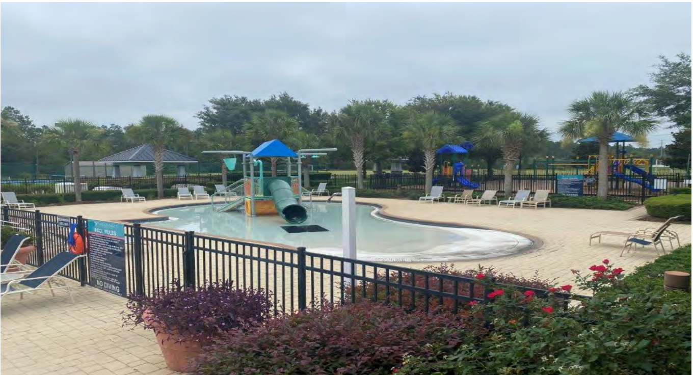
Amenity Center – Kid Pool and Splash Area (Undergoing Repairs) (6-27-23)
