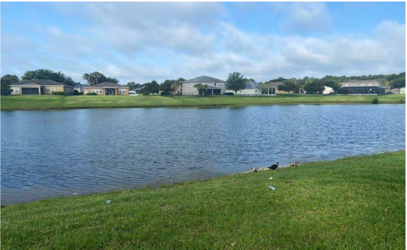
Storm Water Management Facility 2 (6-27-23)
