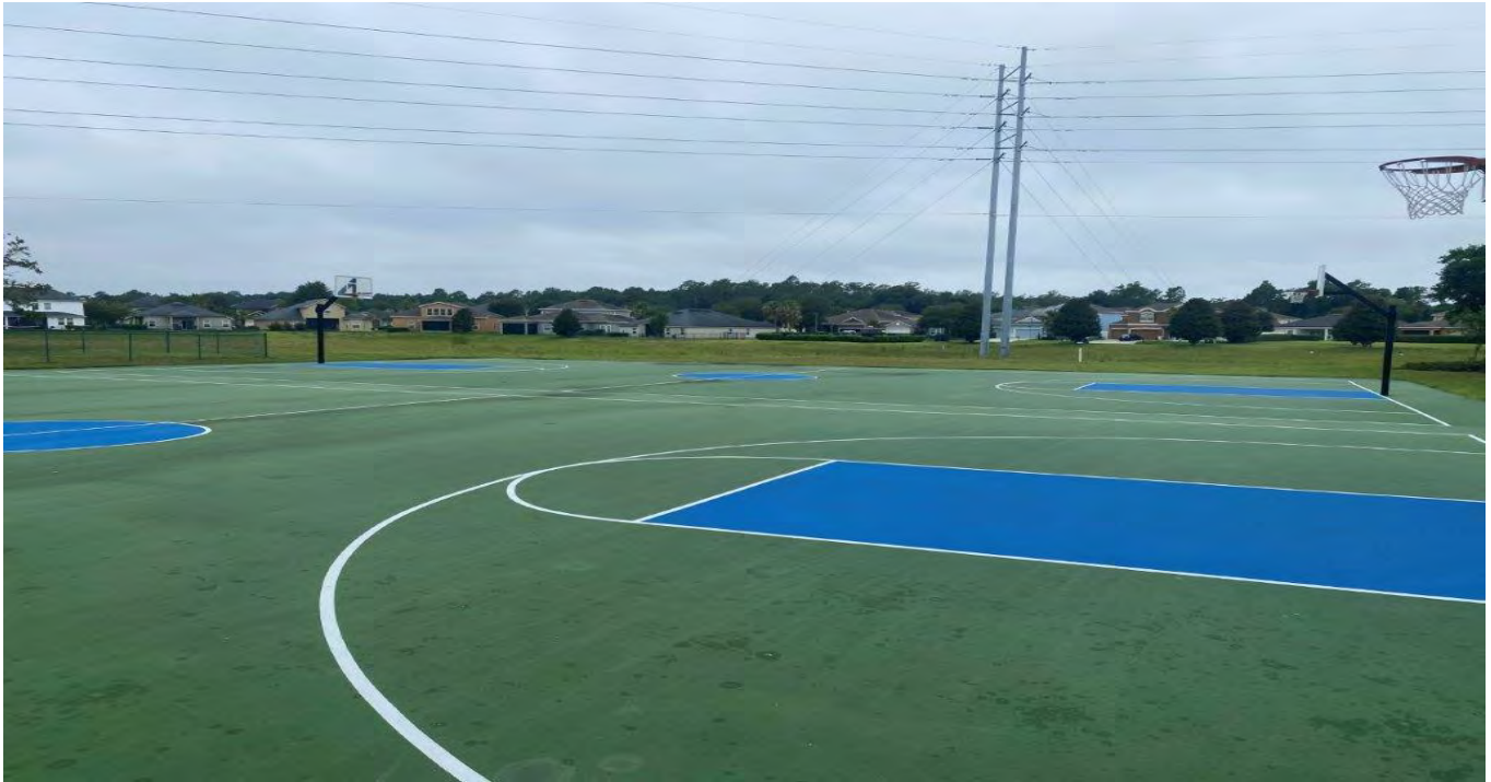
Amenity Center – Basketball Courts (6-27-23)
