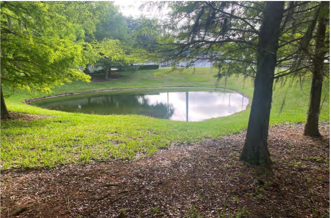
Storm Water Management Facility 9 (6-27-23)
