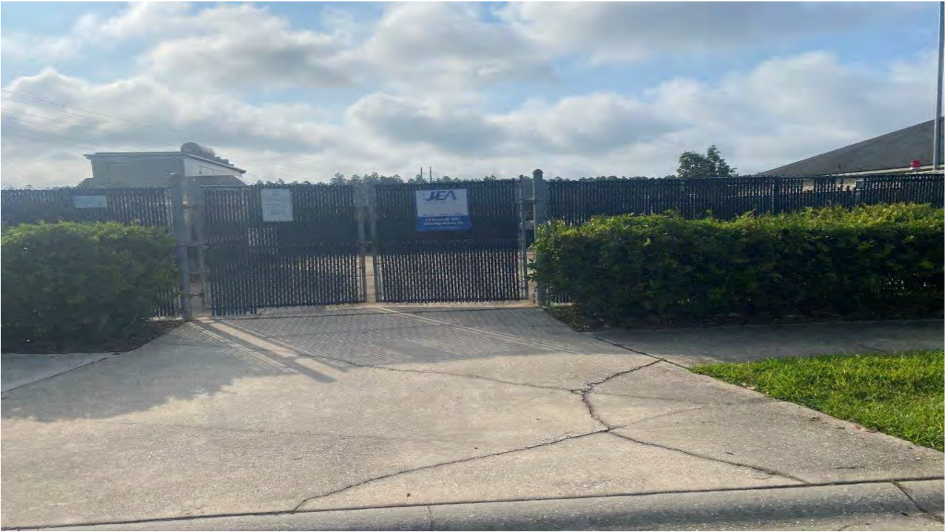
Lift Station – Landscaping (Maintained by the CDD) (6-27-23)
