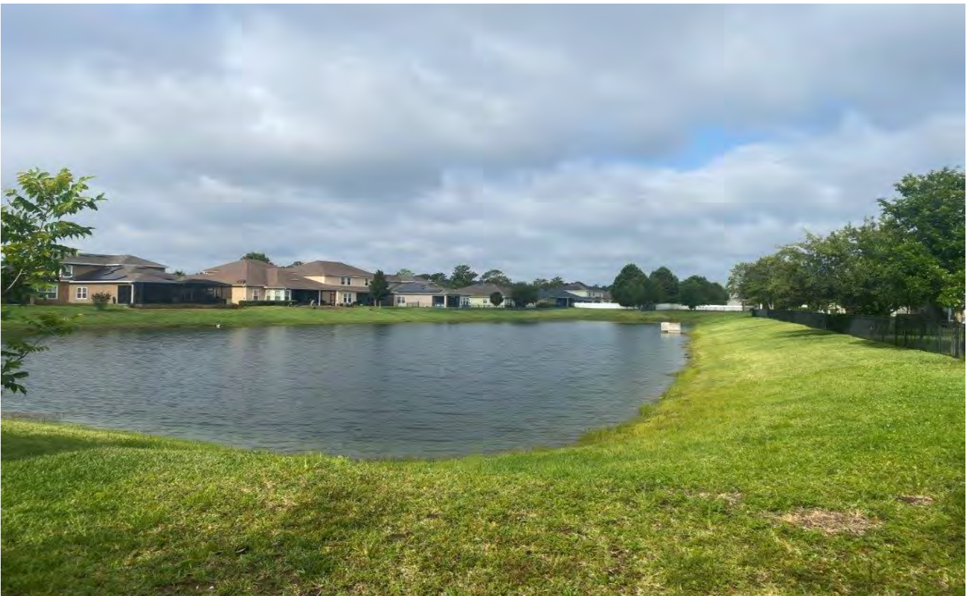
Storm Water Management Facility 7 – Control Structure (6-27-23)
