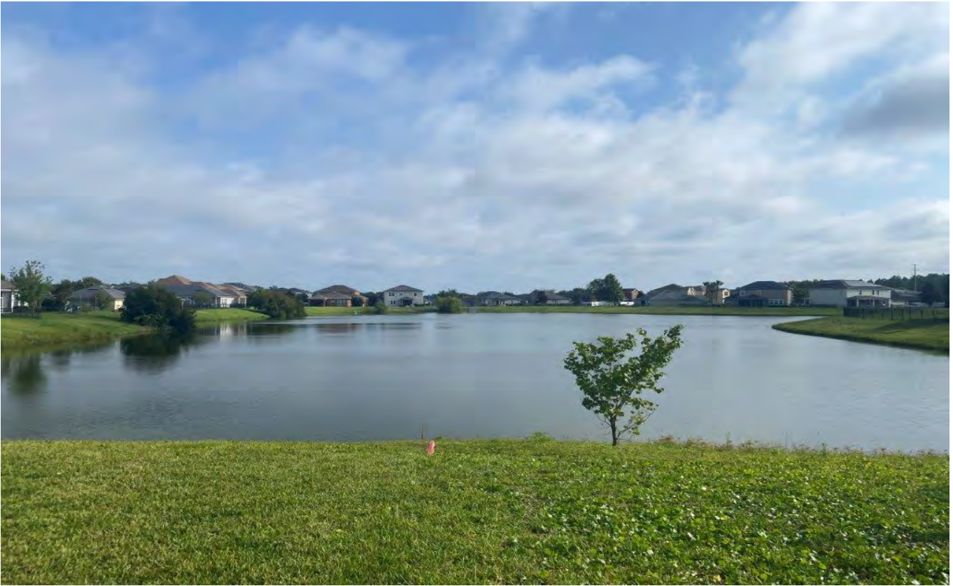
Storm Water Management Facility 5 (6-27-23)
