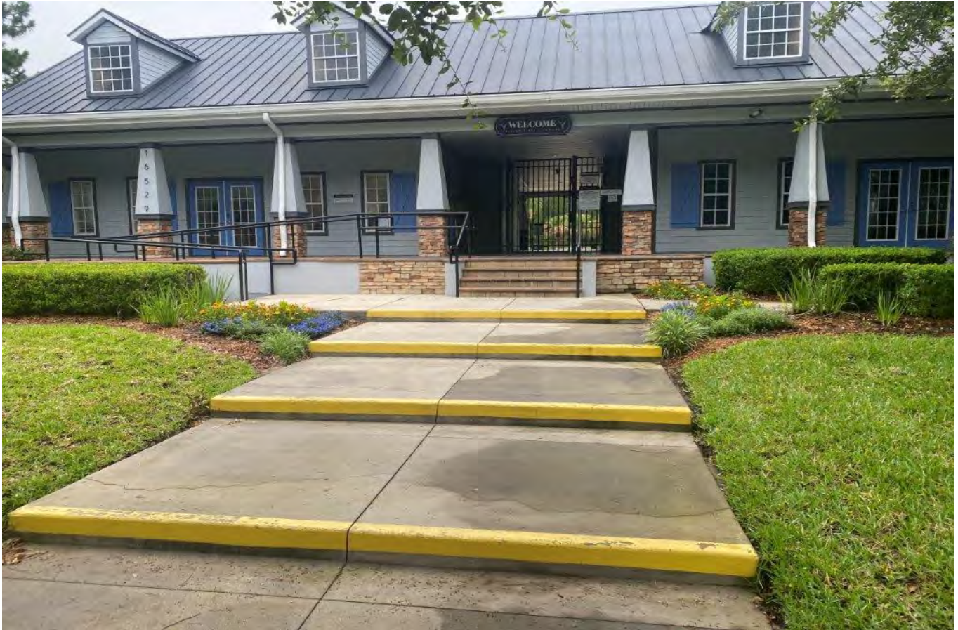
Amenity Center – Front Entrance (6-27-23)
