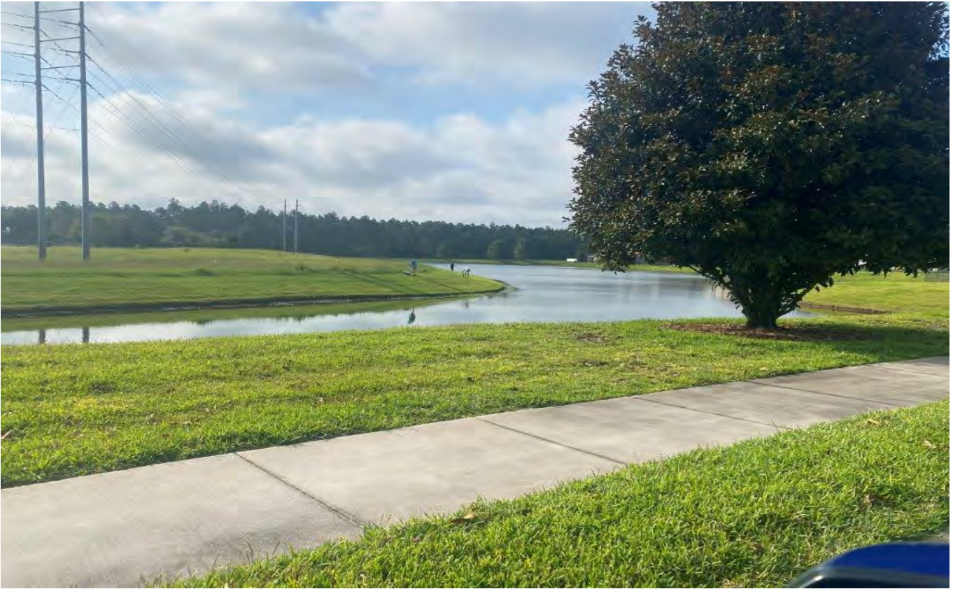
Storm Water Management Facility 1 (6-27-23)
