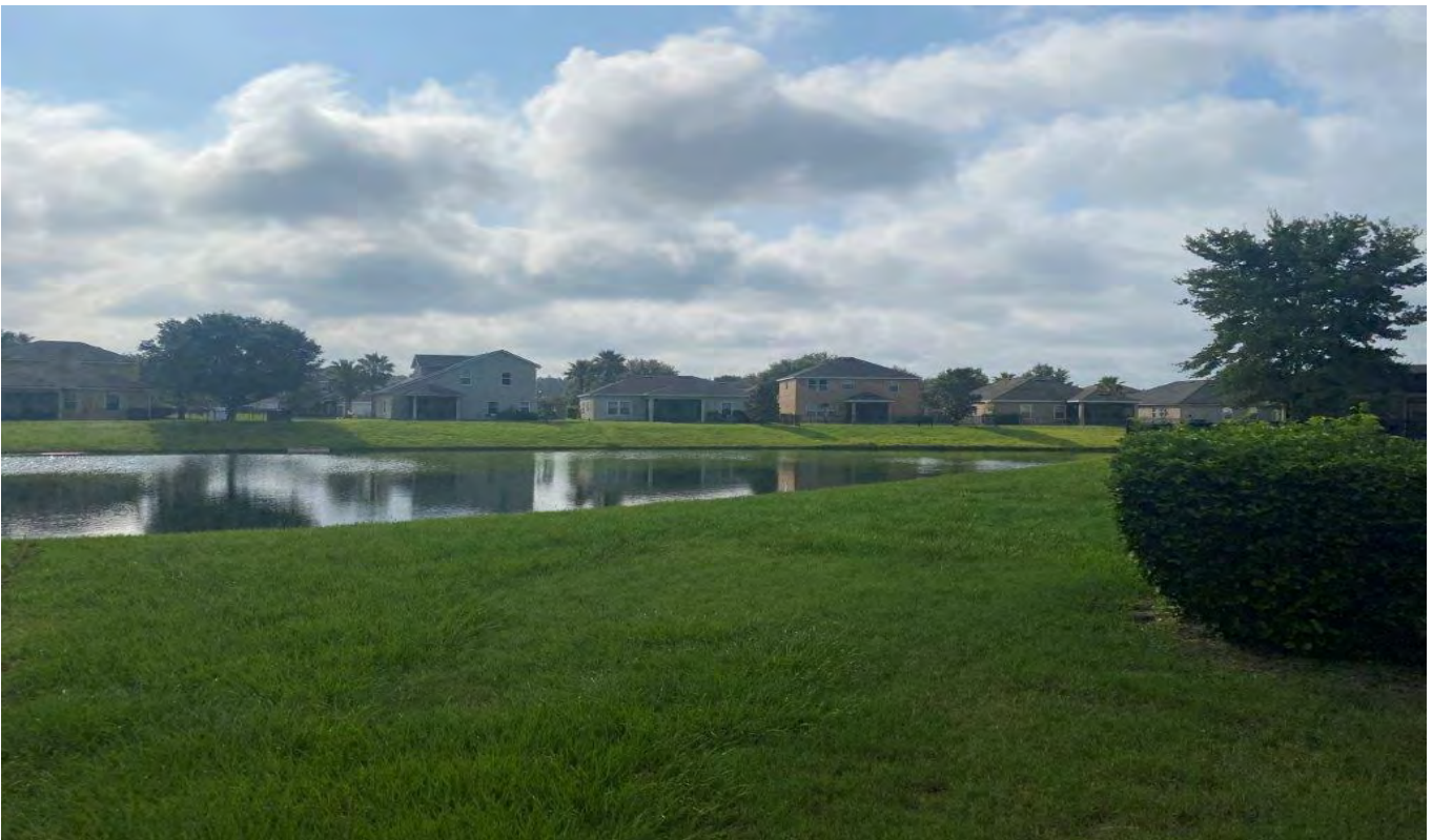
Storm Water Management Facility 4 (6-27-23)
