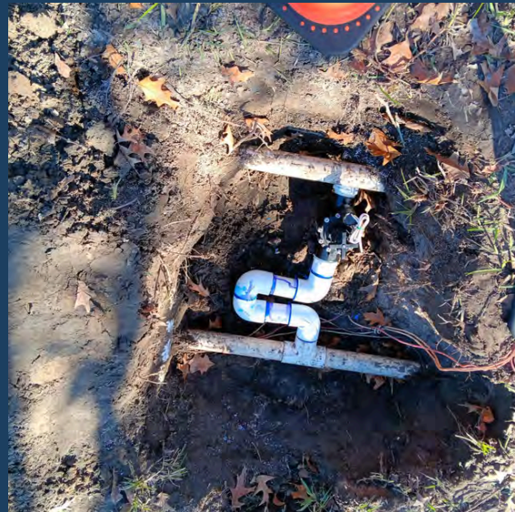
Main St irrigation leak repaired
