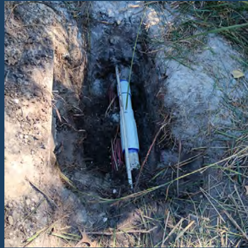
Yellow Bluff irrigation leak repaired
