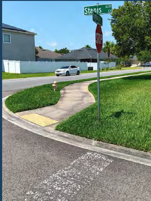
Pic of worn stop bar at Magnolia Grove and Stanis
