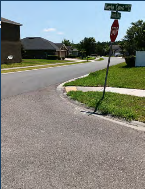
Missing stop bar at Magnolia Grove and Kayla Cove Ct
