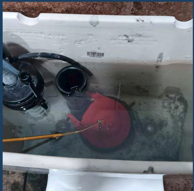
Pic of new flush valve
